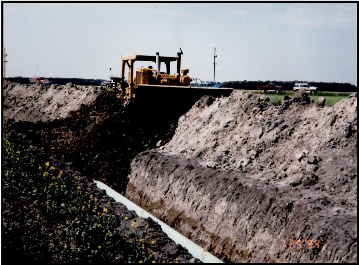
Figure 4.2.7-1 Backfilling
