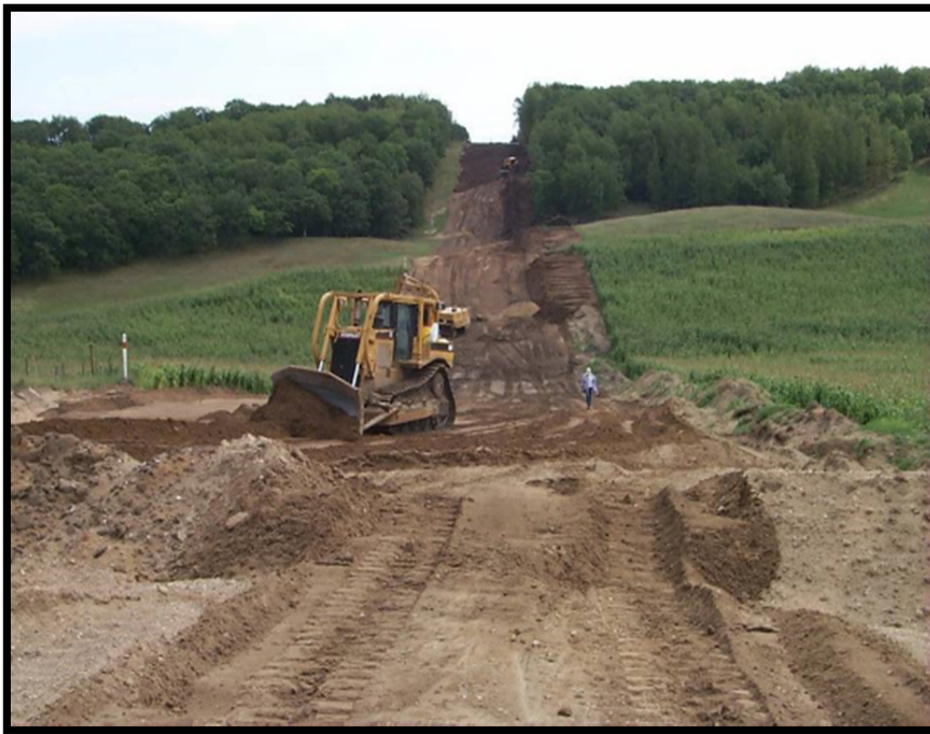
Figure 4.2.9-1 Regrading
