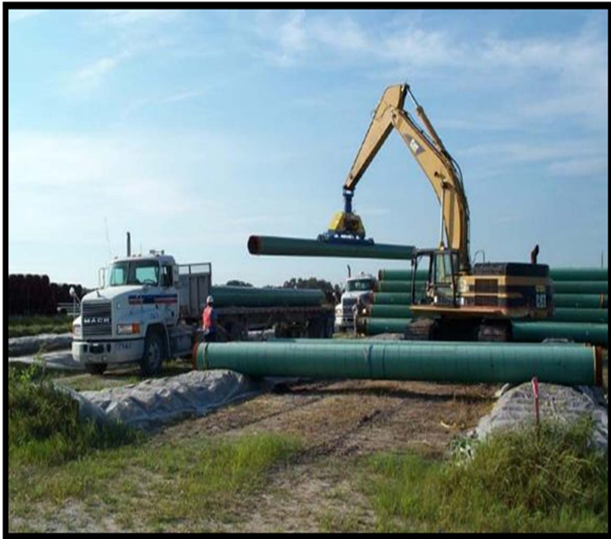
Figure 4.2.4-1 Pipe Loading
