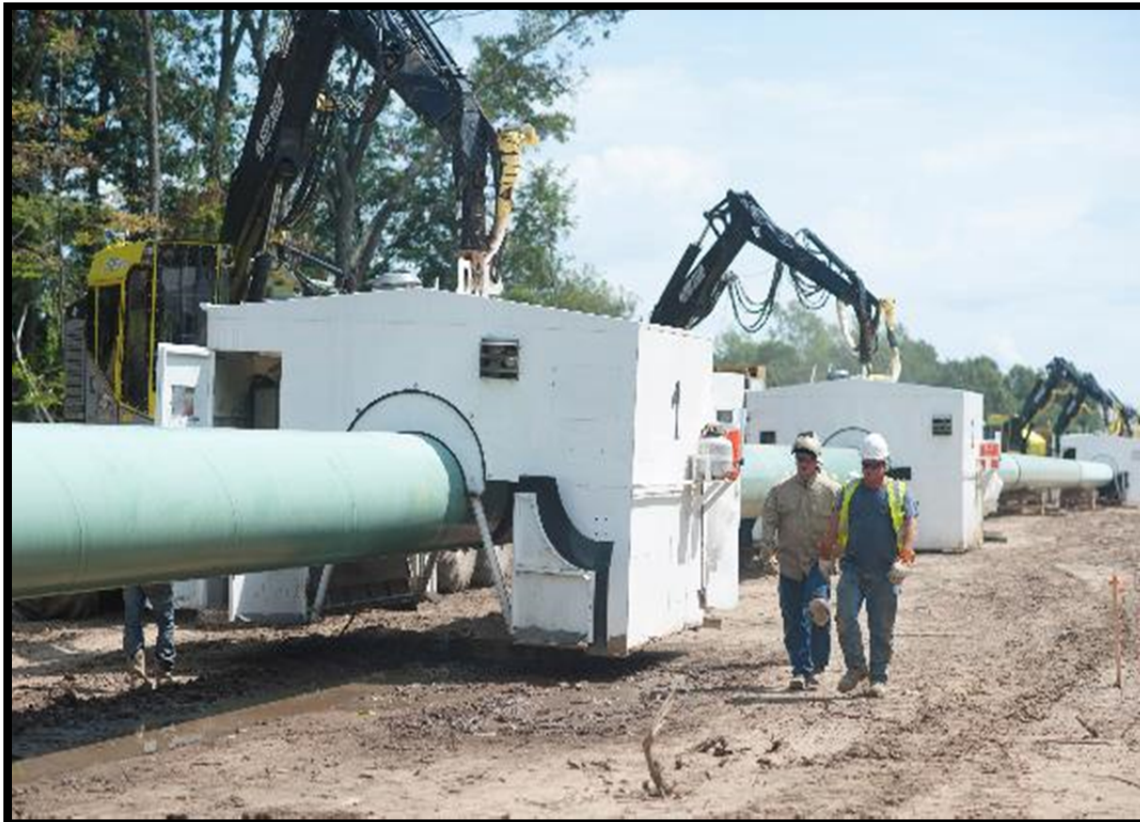
Figure 4.2.5-2 Welding Shacks
