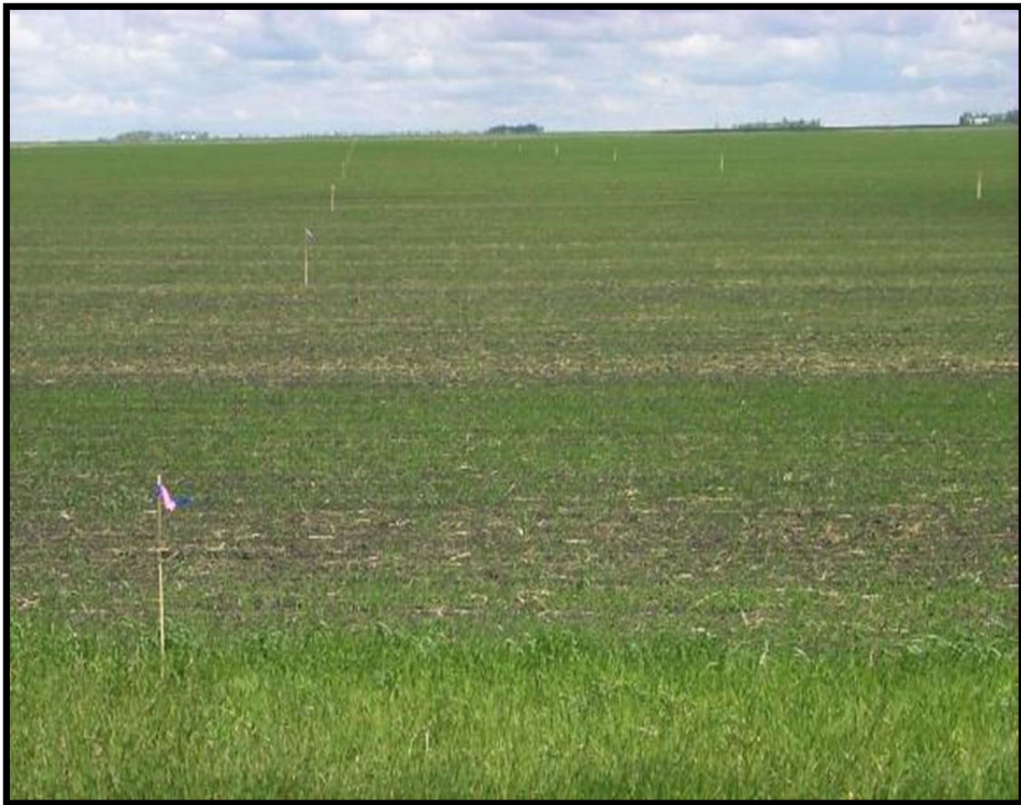
Figure 4.2.1-1 Right-of-Way Staking
