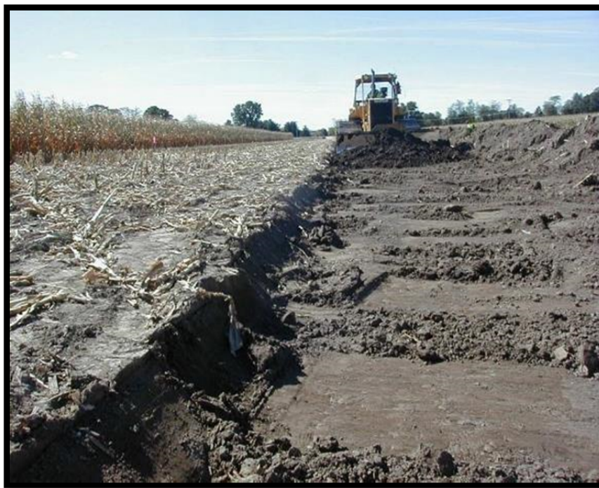
Figure 4.2.3-1 Topsoil Segregation
