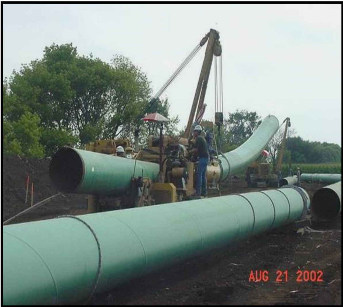
Figure 4.2.5-1 Field Bending
