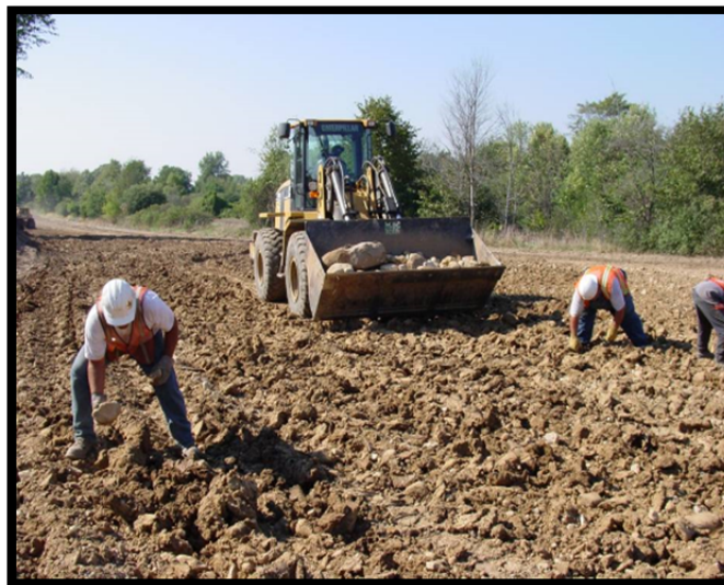
Figure 4.2.9-3 Rock Removal
